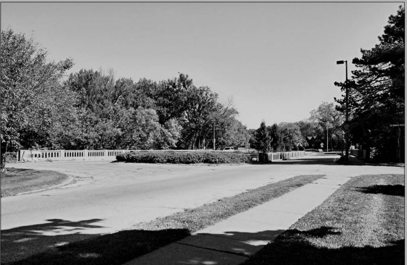
Photo 30 of 31. View from west of Penny Bridge carrying Sheridan Blvd over the Rock Island Railroad (now Rock Island Trail), west of S 33rd. The bridge was built in 1934
