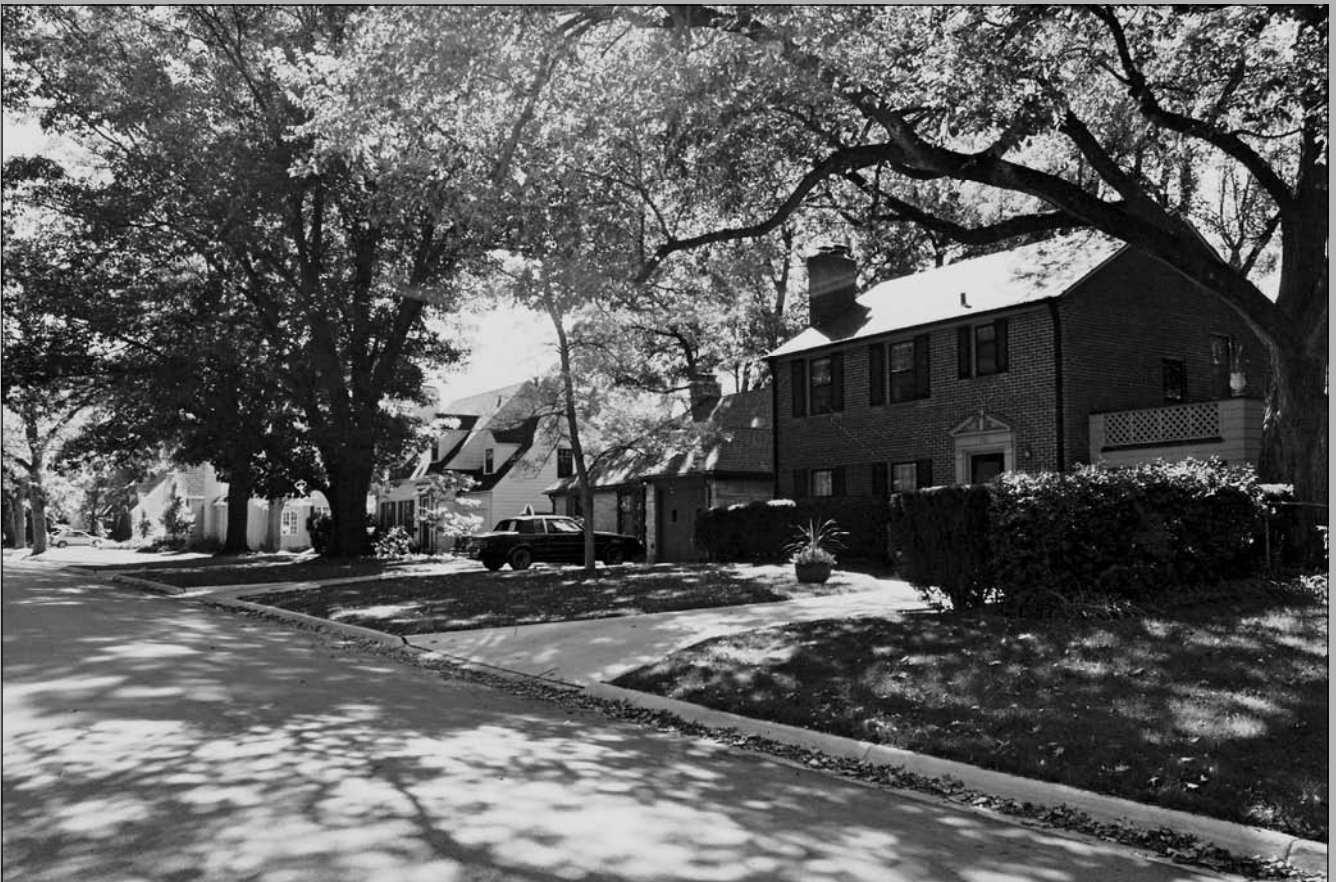
Photo 24 of 31. View from north on S 29th St. 3125 S 29th is at left.
