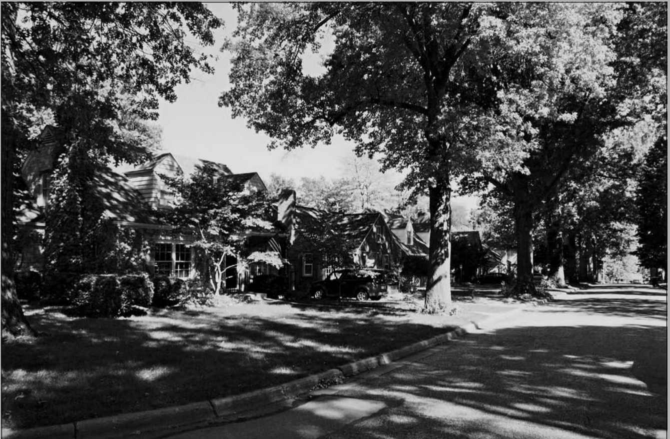
Photo 28 of 31. View from southwest of north side of Alden Ave, east of Winthrop Rd. 3100 Alden Ave is at left, built in 1940
